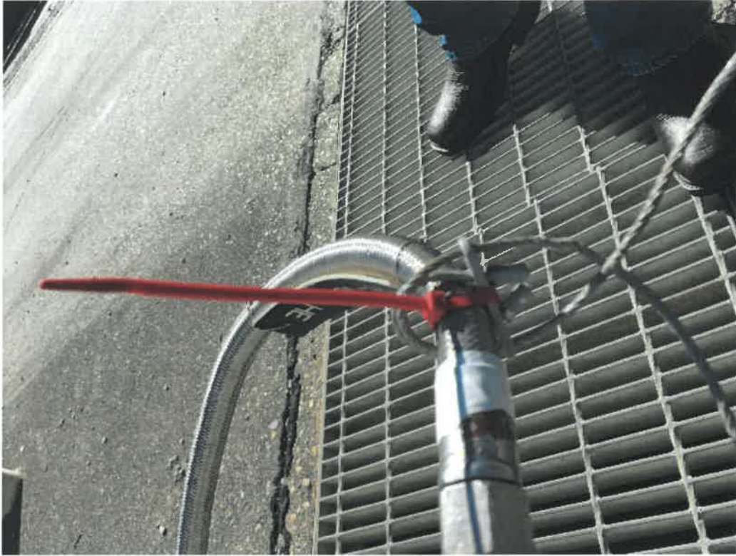
Figure 4. Tie-wrap Installation
